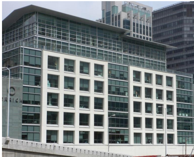
Figure 2. The two four-bay moment frames resist earthquake forces acting along the building. Similar frames are expected to be on the other side of the building.
