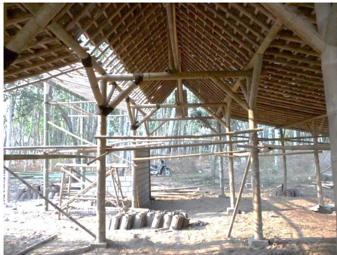
Figure 1. A very flexible building during horizontal shaking. Traditional construction materials and methods are incorporated into a new traditional Indonesian building.
