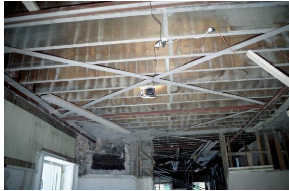
Figure 5. A timber floor of a masonry building is strengthened for earthquake resistance by steel bracing underneath it.
