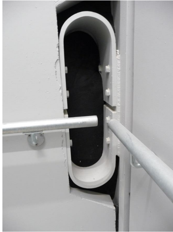
Figure 7. An earthquake energy absorber located between two rocking walls.
