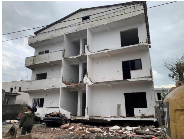
Figure 4. This soft story building lost its ground floor during a moderate earthquake (N. Vesho).
