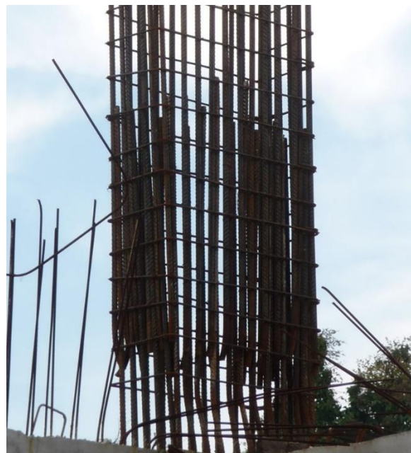
Figure 2. The reinforcement of this column does not comply in numerous ways with the local codes and standards. During a moderate to large earthquake, it will be seriously damaged.
