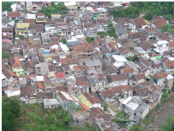
Figure 2. Codes and their implementation are necessary to improve the earthquake-safety of this type of housing.
