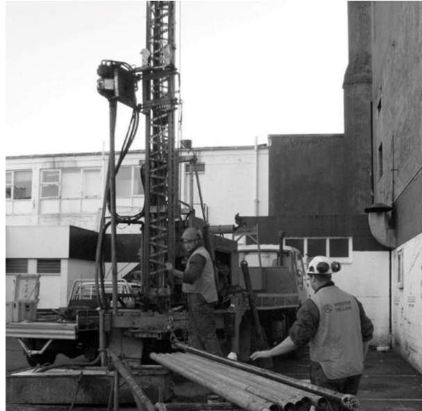
Figure 3. A drilling rig sampling soil to be tested in a laboratory.
