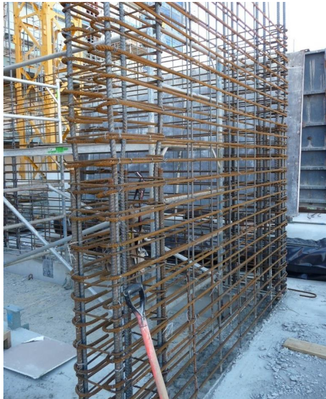
Figure 1. Severe damage during an earthquake could occur if several reinforcing bars are missing from this reinforced concrete wall.
