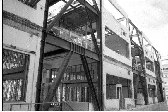
Figure 4. Bays of steel bracing are inserted into this building as part of the retrofit.
