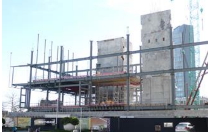
Figure 3. A building under construction. Most of the earthquake forces in both directions are resisted by reinforced concrete structural walls. In this case, some assistance is also provided by a perimeter steel moment frame.
