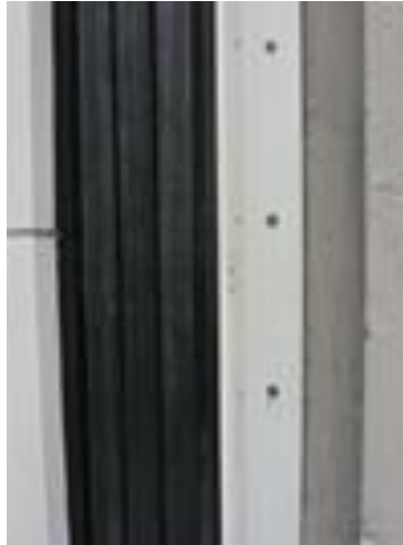
Figure 5. A close-up of the flashing covering the seismic gap.
