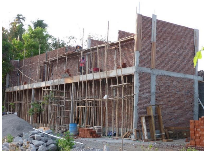
Figure 3. Conventional heavy construction using reinforced concrete and masonry - in this case, confined masonry construction.
