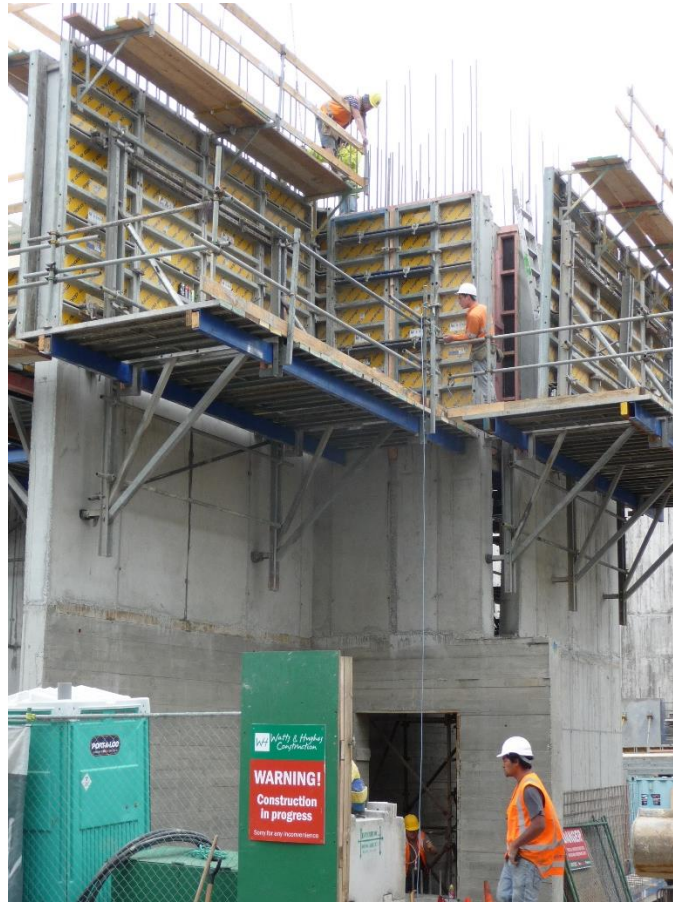
Figure 2. During both design and construction these reinforced concrete walls were checked by engineers to ensure the structural design was sound and that construction was in accordance with the plans.
