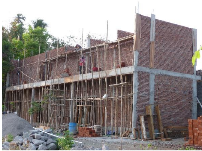
Figure 2. A confined masonry house under construction.
