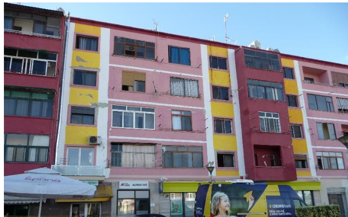
Figure 1. People expect to live in buildings that are safe in earthquakes.
