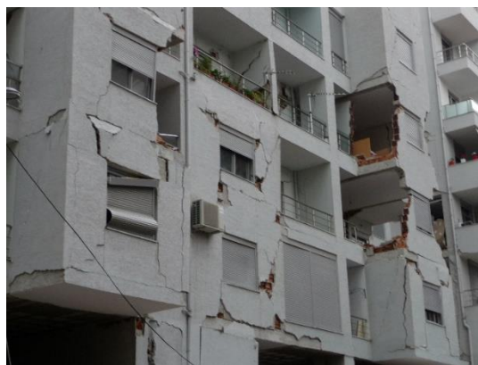
Figure 2. Earthquake-damaged infill walls, some of which have fallen out of the building.
