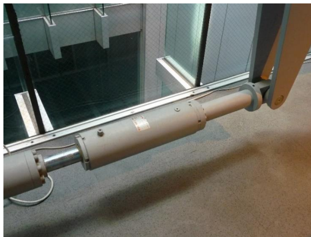
Figure 3. A damper to reduce earthquake movements.
