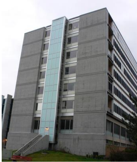
Figure 2. The seismic retrofit of this hospital building included two new structural walls and foundation at each end.
