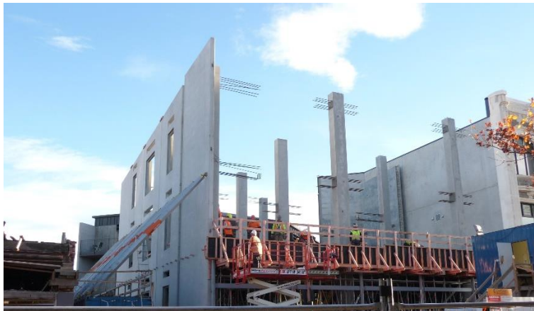
Figure 2. This building contains innovative examples of the use of precast concrete.
